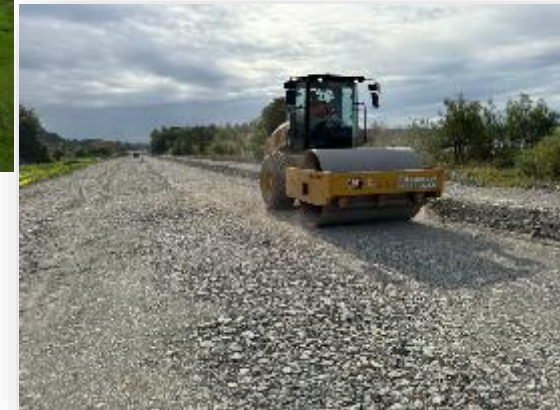
Construction of spine road embankment
