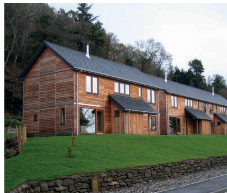
Eachaig, Kilmun Development of 4 affordable houses delivered by Fyne Homes Housing Association as shared equity
