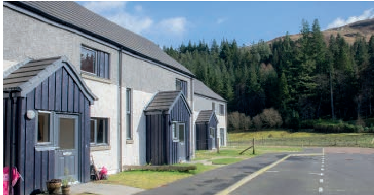
Highland Drive, Lochgoilhead Development of 18 houses delivered by Dunbritton Housing Association
