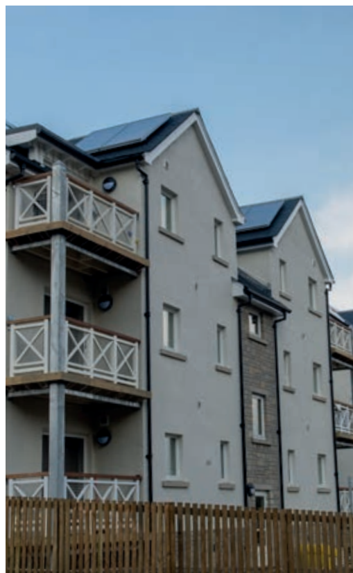
Main Street , Killin Development of 12 social rented flats provided by Stirling Council
