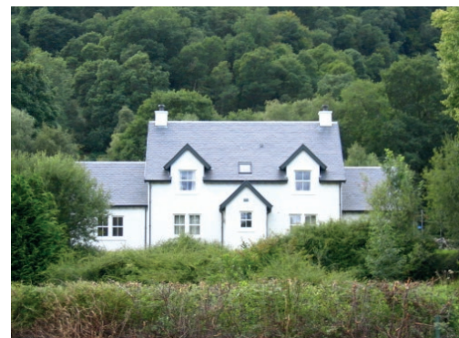
Stonvar, Balquhidder Replacement house
